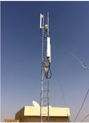
Figure 2: An LTE Advanced base station with three tower-mounted remote radio heads used for broadband wireless.
