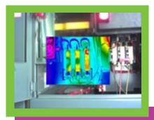
Fluke thermal imagers now include IR-Fusion<sup>™</sup>\*, a technology that fuses a visual, or visible light, image with an infrared image for better identification, analysis and image management. The dual images are accurately aligned at any distance heightening details so problems are easier to spot. \*The Fluke Ti20 comes with InSideIR<sup>™</sup> analysis and reporting software with free updates for the life of the product.
