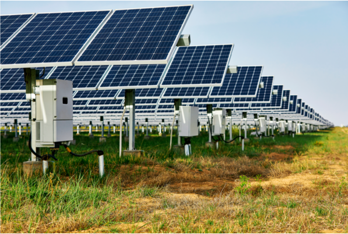
Figure 1. Inverter boxes connected to photovoltaic panels.
