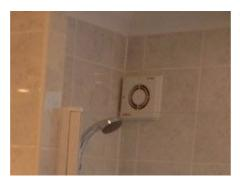
The illustration shows a duct fan in a typical installation as found in bathrooms and toilets in private buildings and hotel rooms and sanitary rooms in catering establishments. Only the fan guard can be seen from outside, the fan itself and the electrical connection is concealed in the wall.
