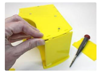
Insert the "roof" of the cabinet. The roof and back pieces are similar in size, but the tabs are spaced differently, so only the correct piece will fit.
