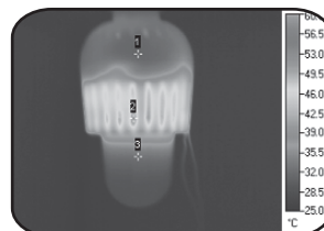
IR thermograph inspect
