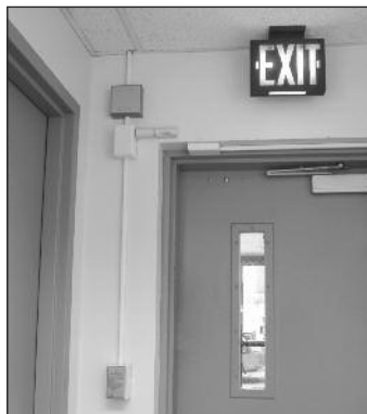
Typical applications for 500 & 700 Series Raceway.
