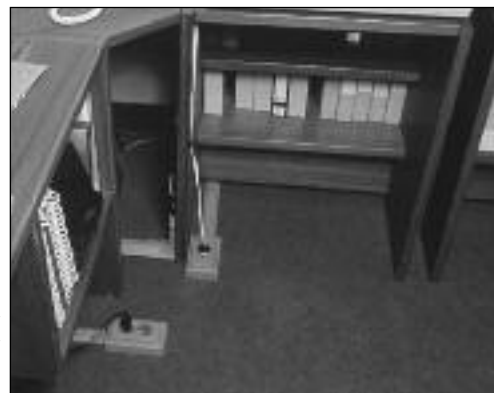
1500 and 2600 Series Overfloor Raceway can be installed over floor coverings to provide either permanent or temporary access to services.
