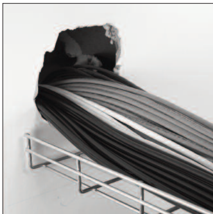
1. Existing hole with cables. Irregular hole cut.
