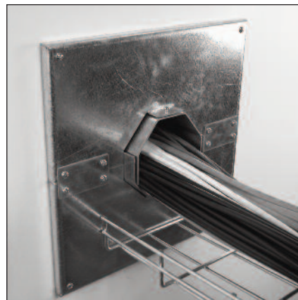
3. Push split conduit into wall.
