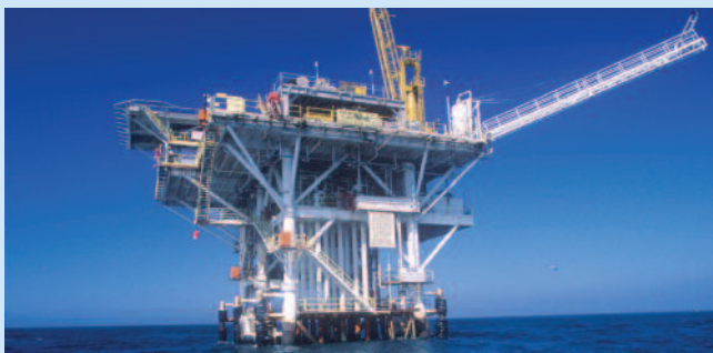
Offshore / Civil Marine
