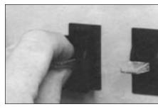
Replace lever assembly and "snap" escutcheon into place. Installation complete!
