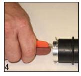
Step 4: Remove clear poly interlayer by slitting each end of the tape longitudinally away from the jacket to the end of the cable. Use the inner jacket as a guide to remove each piece of the poly. Do not cut into inner tape. The inner shield will now be fully exposed.
