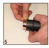
**Step 6:** Apply adhesive copper tape completely around the cable core shields. Both inner and outer shield will be in full contact with tape. Both drain wires will be outside the copper tape.
