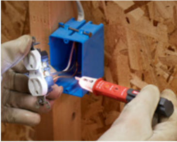
Test wires for AC voltage
