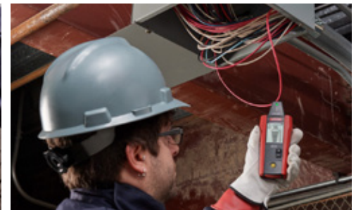
Locate a specific wire
