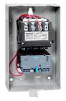
Non-reversing motor starter Size 00 Three phase full voltage Solid-state overload relay OLRelay amp range 3-12A 380-440/440-480V 50/60HZ coil Combination type Indoor general purpose use
