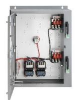
Pump control panel, Duplex controller NEMA size 2 Solid-state overload relay, OLR amp range 13-52A, 120 VAC coil, Fusible disconnect HOA Sel Sw. and Start P.B., Enclosure NEMA type 3/3R,12 Weather proof outdoor use
