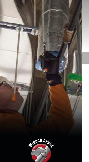
Wrench assist shaft allows for greater torque.
