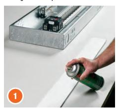
Cut the 3M™ Interam™ Endothermic Mat to fit the sides, top, bottom and back of the utility box. Apply 3M™ Super 77 Multipurpose Adhesive to the box surface and each piece of mat. Let the adhesive dry on the box and mat surface for approximately 1 minute. See UL System W-L-7190 for overlaps and complete system details.
