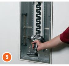
Insert the utility box into the opening so the box is flush with the surface of the wall. Secure the steel box to the steel studs per the utility box manufacturer's installation instructions.
