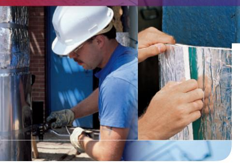
Installing multiple layers of 3M™ Interam™ Endothermic Mat flexible wrap allows you to tailor the desired amount of fire protection—up to 4 hours for structural steel.
