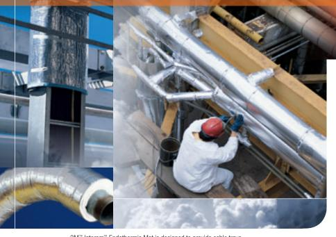
3M™ Interam™ Endothermic Mat is designed to provide cable trays and conduits with full envelope protection in the event of a fire.
