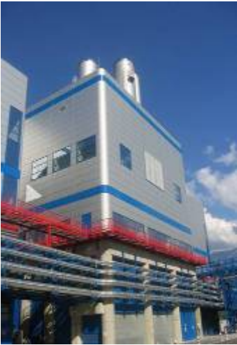
Process exhausts 580 000 m 3 /h
