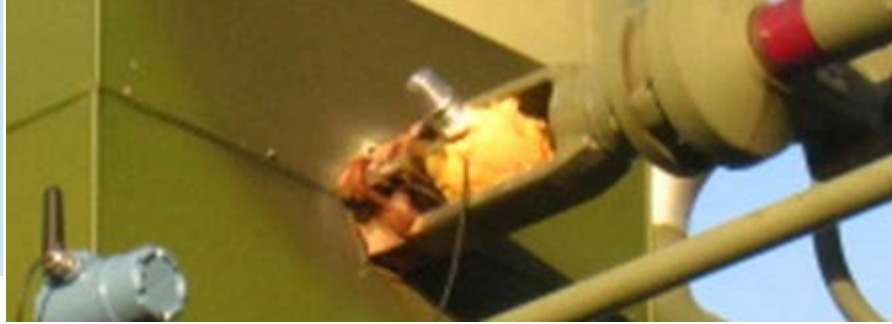
Location for thermoharvesting field test at Shell facility power for wireless sensor devices.
