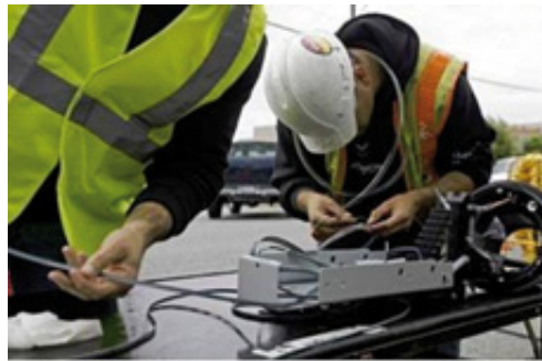
Figure 2 Field fiber splicing
