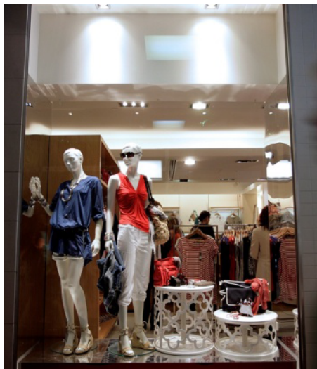
Recessed downlighting in commercial buildings
